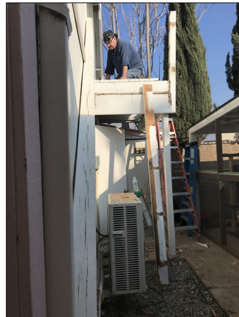
Old stairs and decking coming down.
